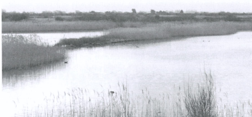
Plate 5 Weston Sewage Treatment Works, North Somerset. View from the north-west across the UV Lagoons. (Photo: Lyndon Roberts)
