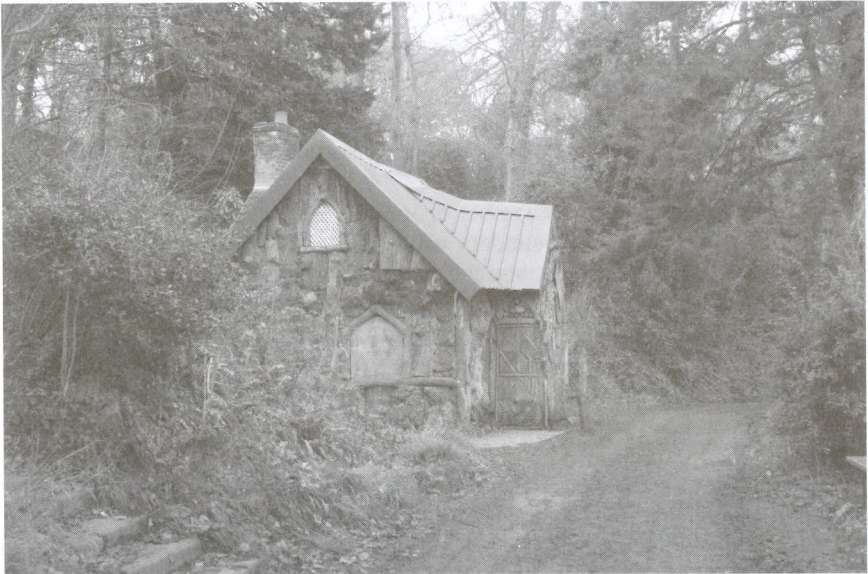
Plate 1 The Timber or Inner Lodge in Blaise Woods, which is undergoing repairs (the roof is normally thatched). The timber cladding of the building provides ideal nest cavities for tits Paridae and Treecreeper Certhia familiaris .
